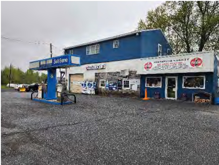
Commercial building and dispensers looking southwest
