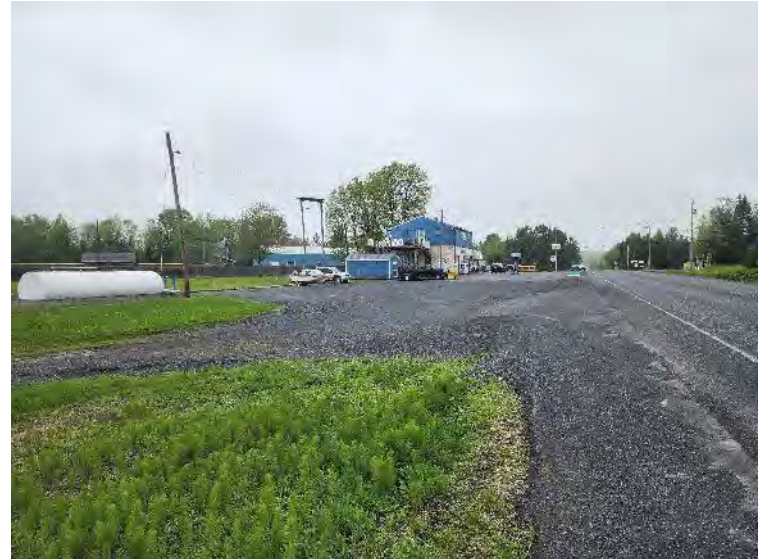
View of subject property looking northwest, Route 161
