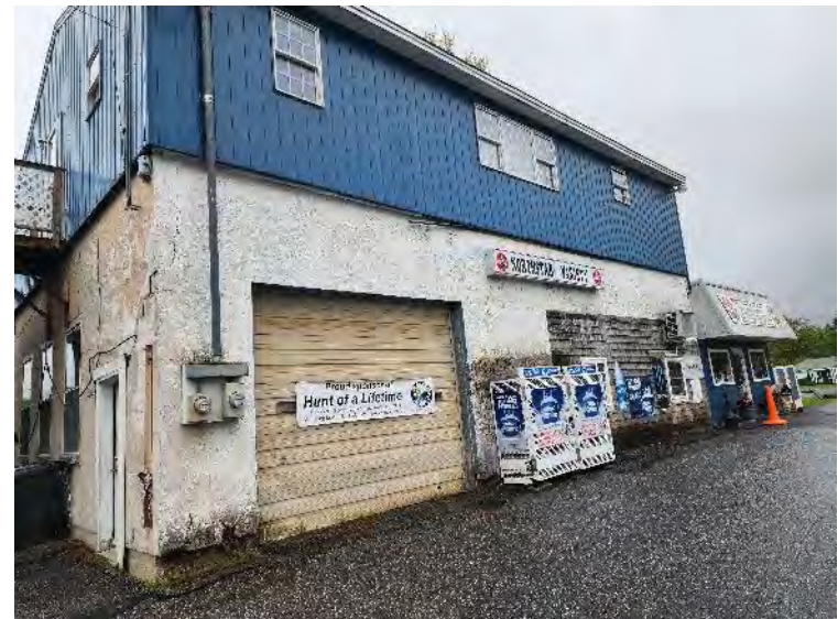
East side of commercial building looking northwest, garage
