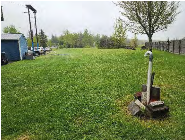
Vent pipe, holding tank west of commercial building
