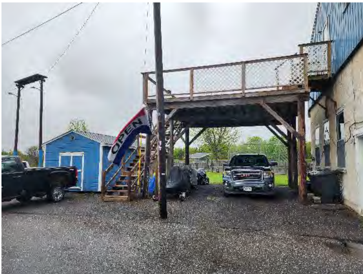
Shed, deck, trash bins, fill and vent piping south of commercial building
