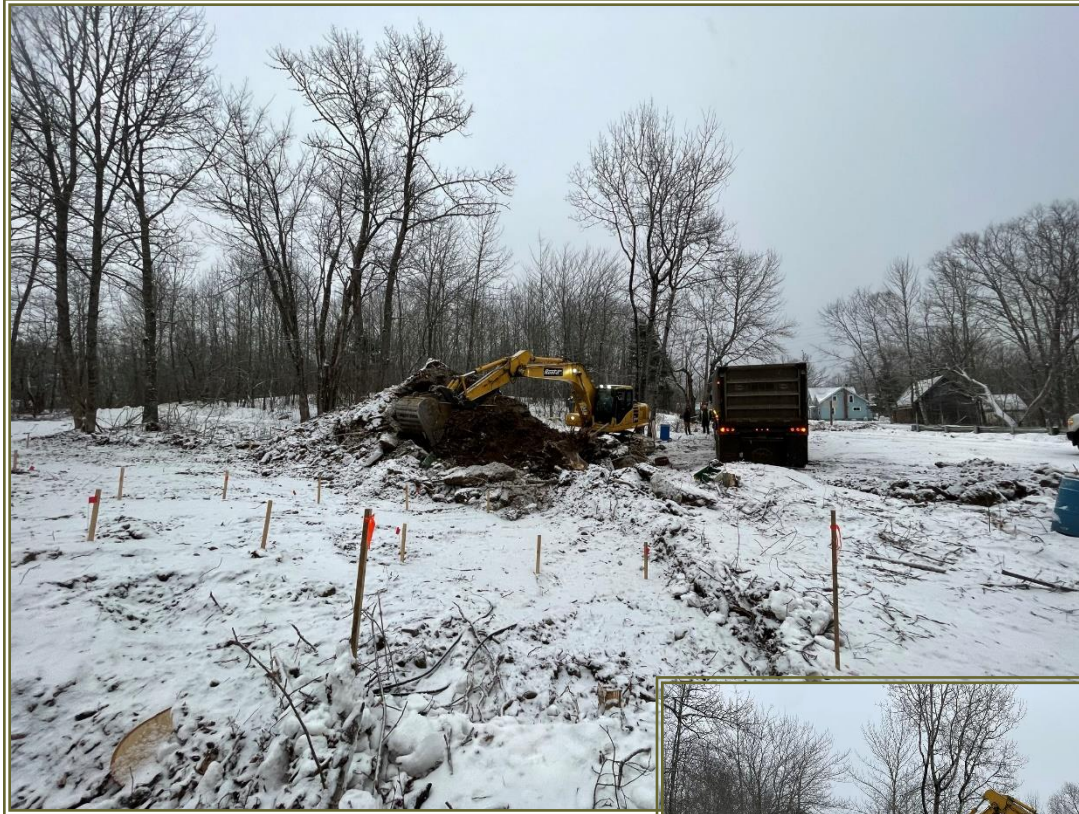
Removing PCB-impacted soil for off-site disposal
