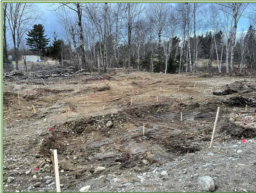
Confirmation Soil sampling following initial excavation
