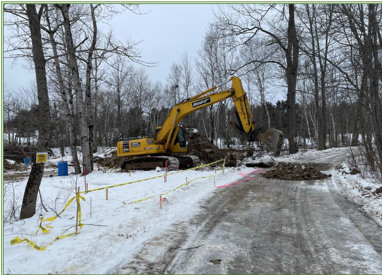
Excavating PCB-impacted soil and using clean fill to repair the driveway
