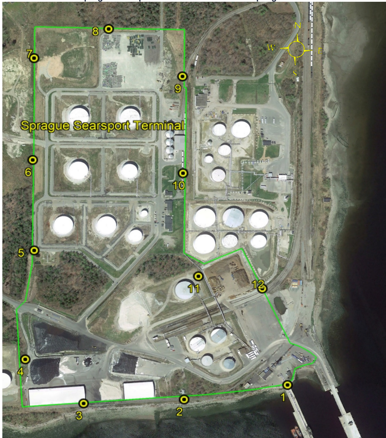
Aerial View of the Sprague Seaport Terminal Fenceline Sampling Locations
